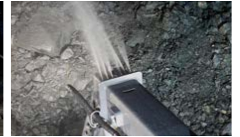
The water sprinker system provides efficient dust control.
